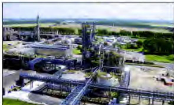
ThyssenKrupp Uhde has built a 3,500 t/day urea plant for Yara in Sluisdijk, Netherlands
