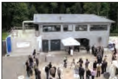
The new treatment plant at the Marienhospital, Gelsenkirchen
